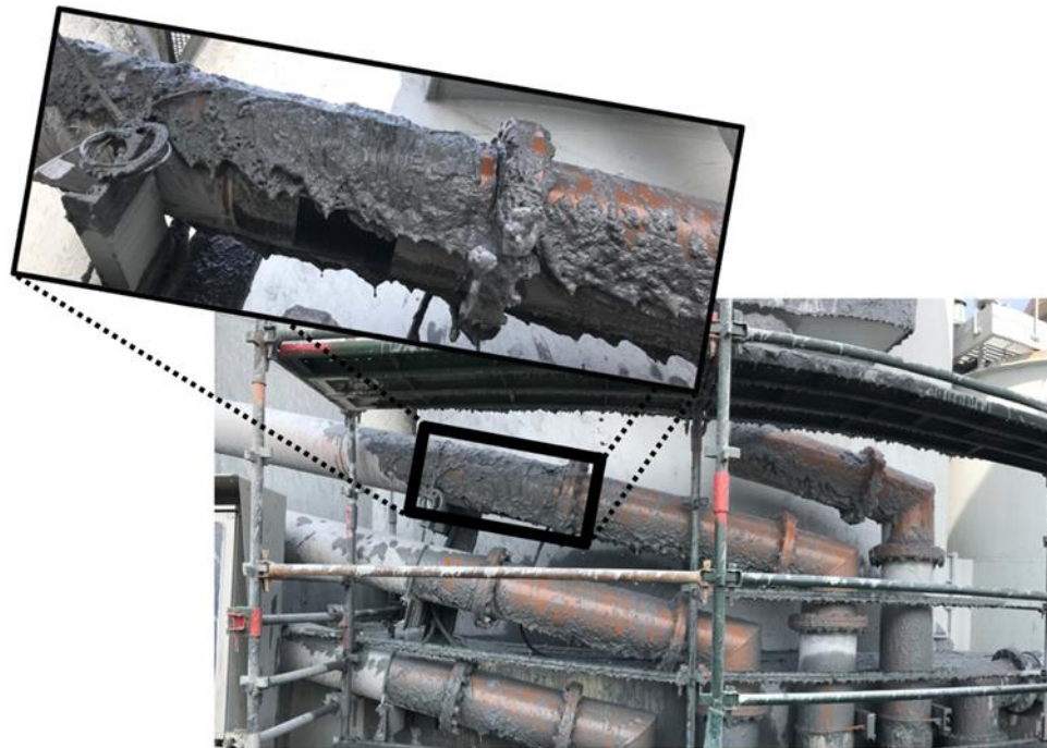
Figure 4: Detailed view of zone 2, the flotation cell concentrate flow metering zone, following installation. Platinum sluff can be seen flowing over the flow meter.
