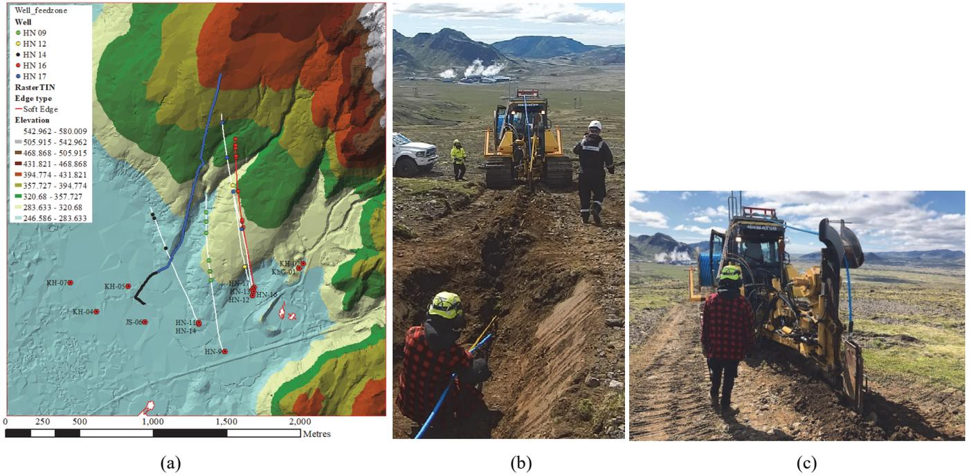
Fig. 5. (a) Location of wells at the Hellisheiði site. HN-16 is the CO<sub>2</sub> injection well. The blue line is the helically wound cable deployment and the black line is the tactical cable joining the HWC to the DAS interrogator, (b), (c) installation of the HWC at the Hellisheiði geothermal site.
