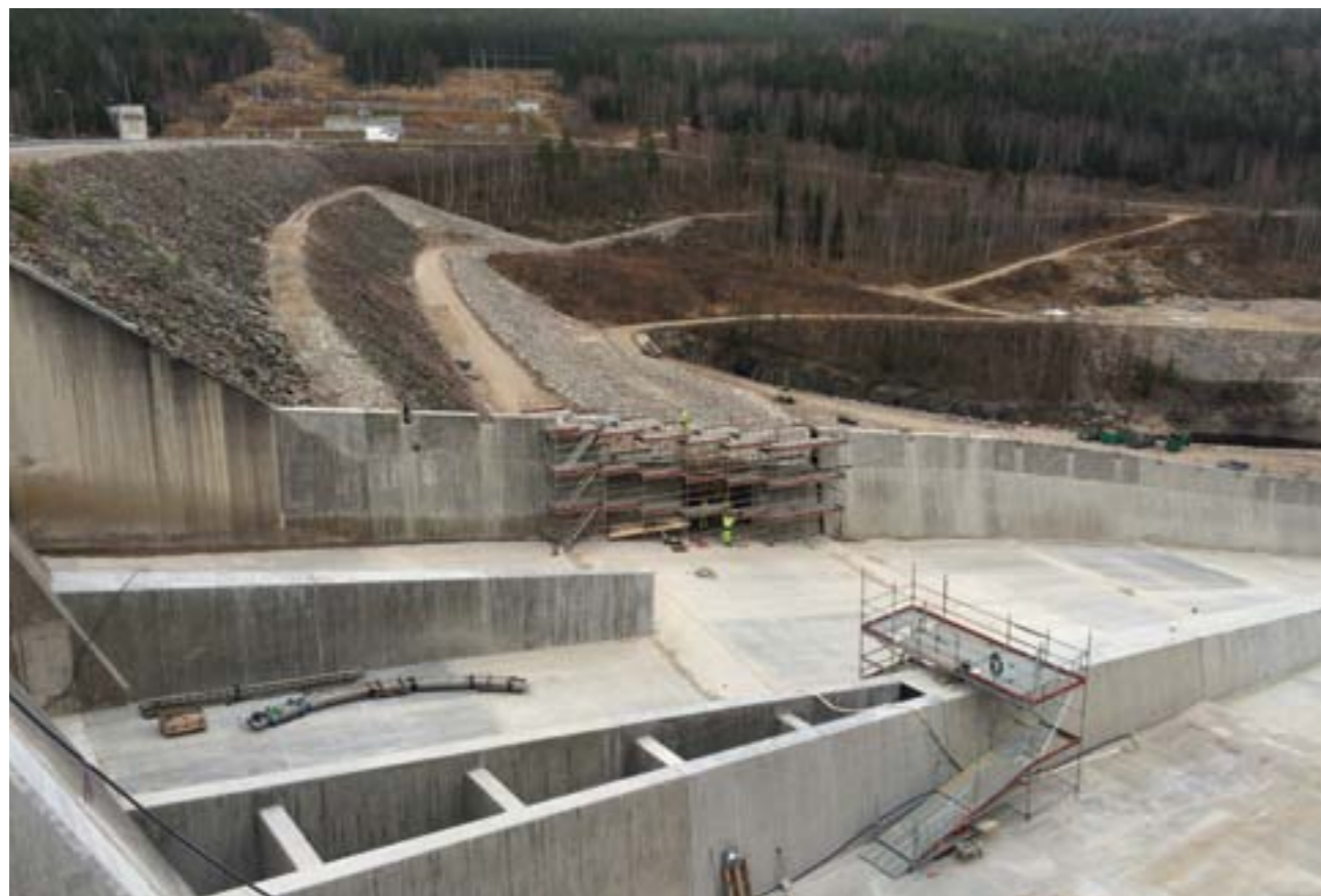
Below: Installation work at Höljes dam
