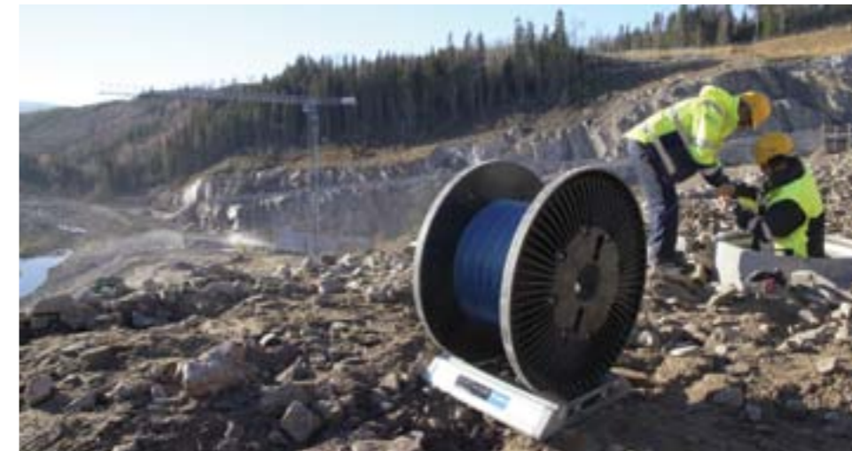
Left: Cable installation at the dam
